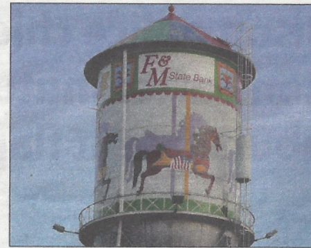
CHRIS LEE/ CHRIS.LEE@ APG-SW.COM Waterloo's "carousel" water tower at 212 Squire St. on June 19.
