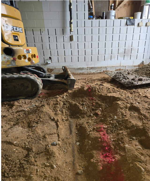
Site Prep for new blower room concrete floor
