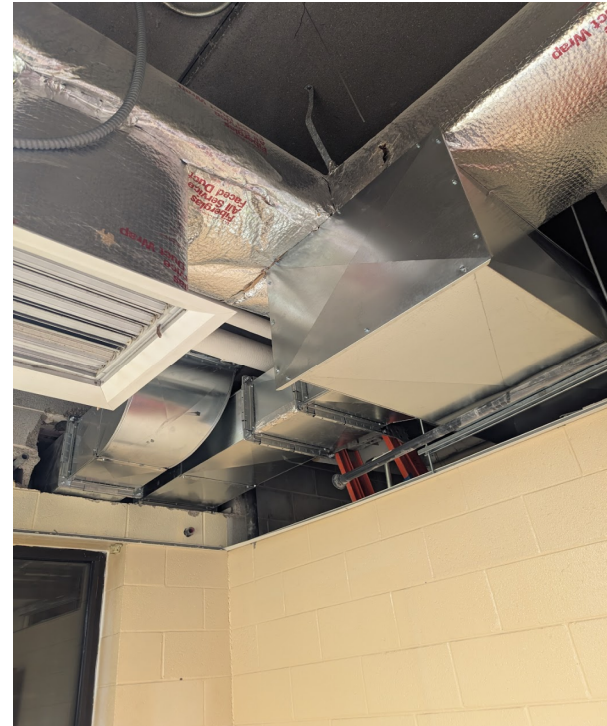
Structure 10 Connecting HVAC to new part of structure
