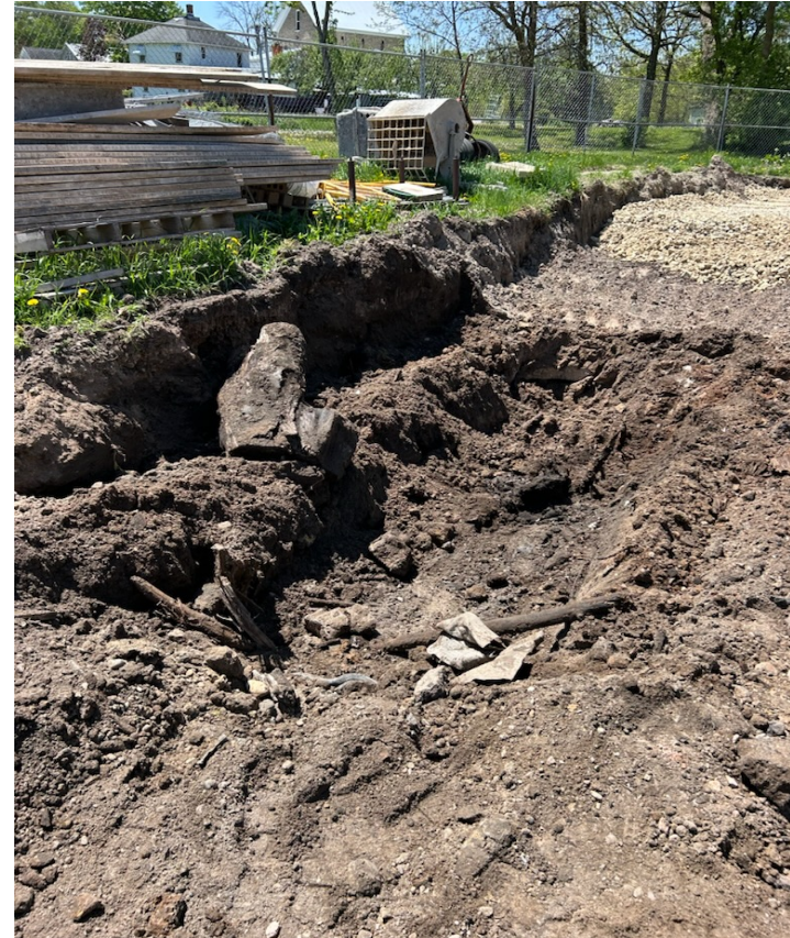
Site Excavating to subbase for asphalt
