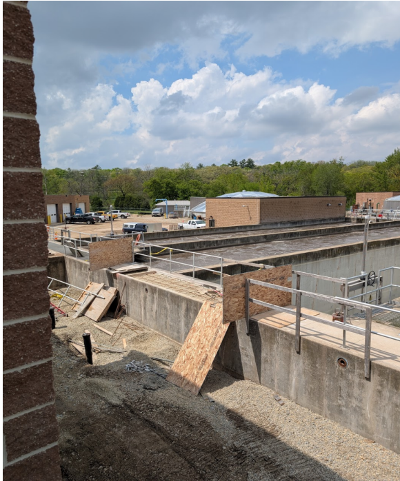
Structure 30 Filling in influent channel
