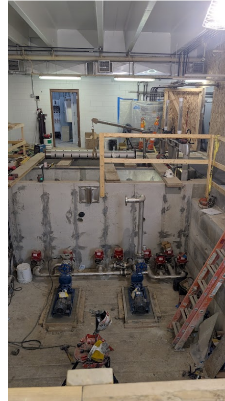
Structure 50 Backwash piping install for Disc Filters 3 & 4
