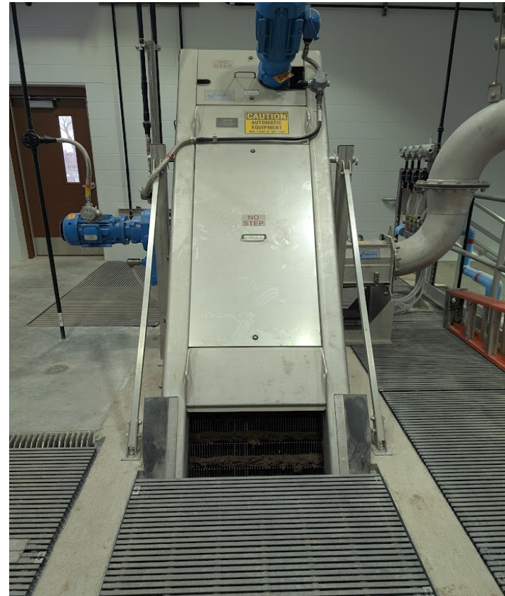
Structure 25 New stair screen filtering influent
