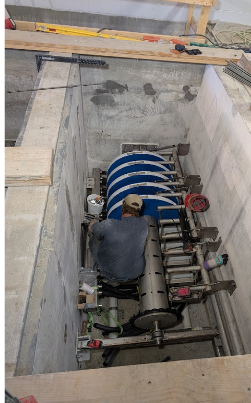
Structure 50 Install of Disc Filter 4
