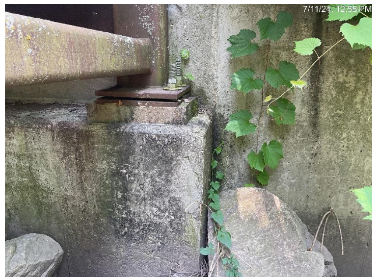
Minor map cracks at West abutment, North bearing
