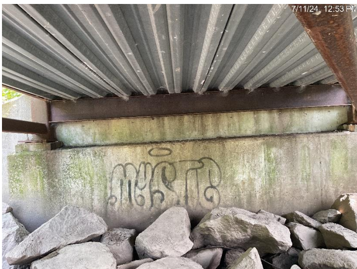
West abutment and floor beam typical condition
