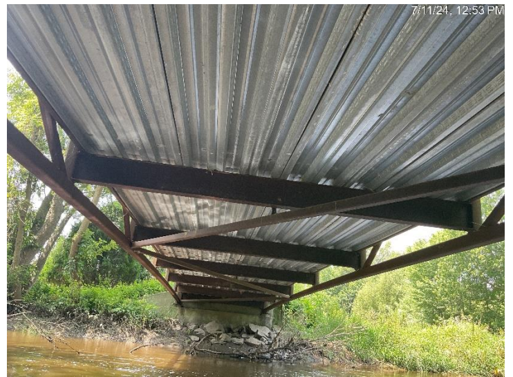
Typical view of SIP and truss lower cord
