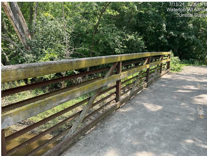
Typical algae growth on rails and truss
