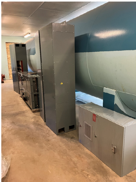
Booster Station - MCC Section and Control Panel Delivered
