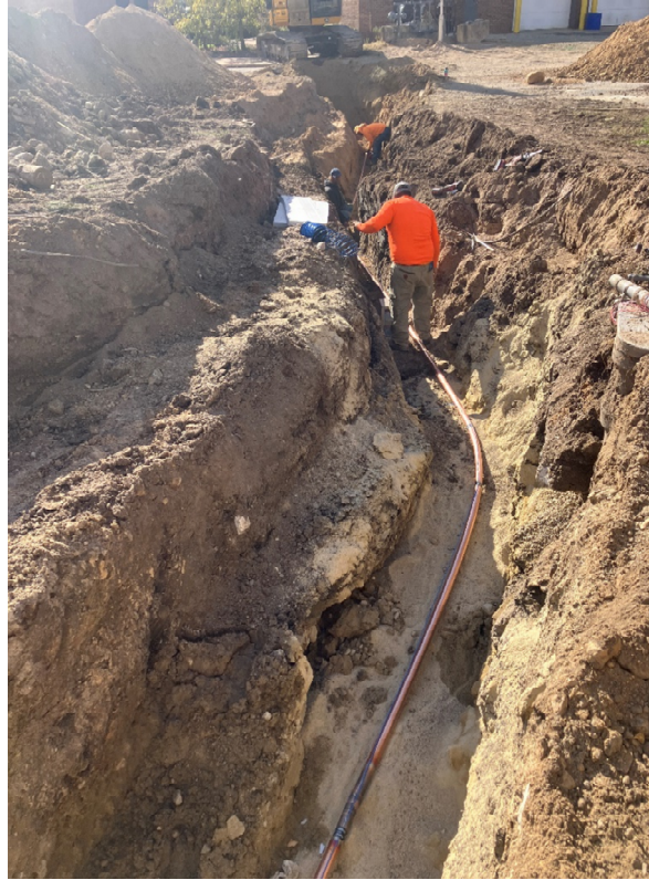
Site 05 - Water line installation
